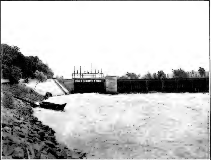
1. The dam in Gruetz on the Havel seen from below; on the right side on the picture the needleweir and on the left side the rampart. Left from it the sloping wall and on its upper edge the trap. (Photographs by Dr. Roehler.)
